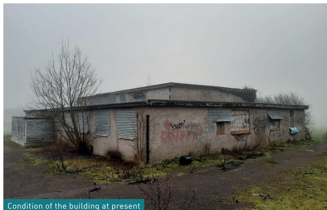
Condition of the building at present
